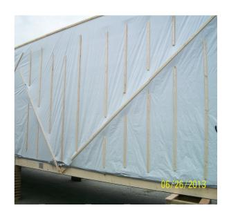
resistance and water resistant product. The proSeal Building wrap is 12' wide and packaged in to length you require for easy installation.
